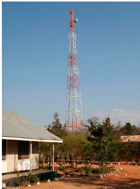
Telecommunications arrive – the tiGo cell phone tower looms large over the new Senior classrooms.
